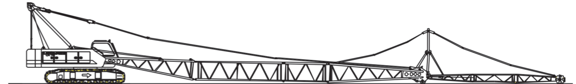
Assembling the boom and anchoring rods
